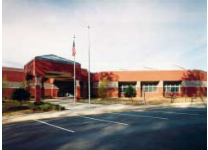
Fig. 1 Durant Road Middle School saves the district $21,000 annually.
