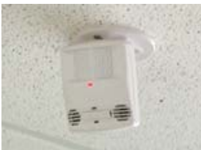
Watt Stopper DT-200 energy-saving motion and light sensors are installed in the classrooms.
