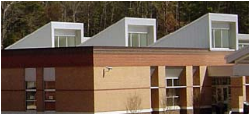
Triangular-shaped roof monitors provide most of the daylighting within the classrooms.
