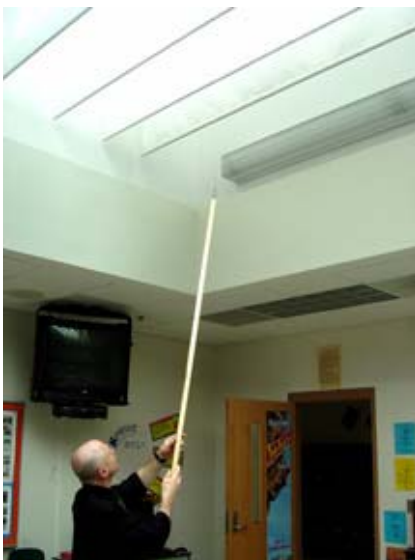
Manually operated vertical blinds on the roof monitor windows can be drawn to darken rooms for audio-visual presentations.
