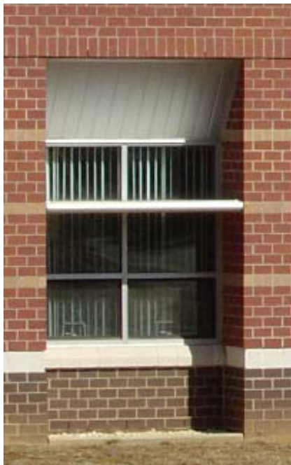
Light shelves and angled soffits maximize and redirect daylight upward through the windows to light-colored ceilings.
