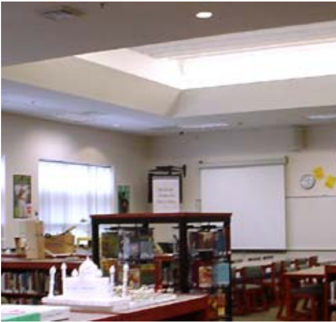
The media center supplements daylighting with recessed and wall-mounted T8 fluorescent luminaires as well as CFL downlighting.
