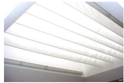
Fabric baffles help ensure uniform light distribution while eliminating potential glare from the roof monitors.
